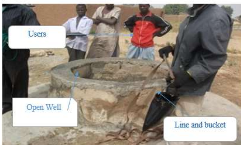
Figure 7.11: Uncovered community HDW with line and rubber drawer being used
