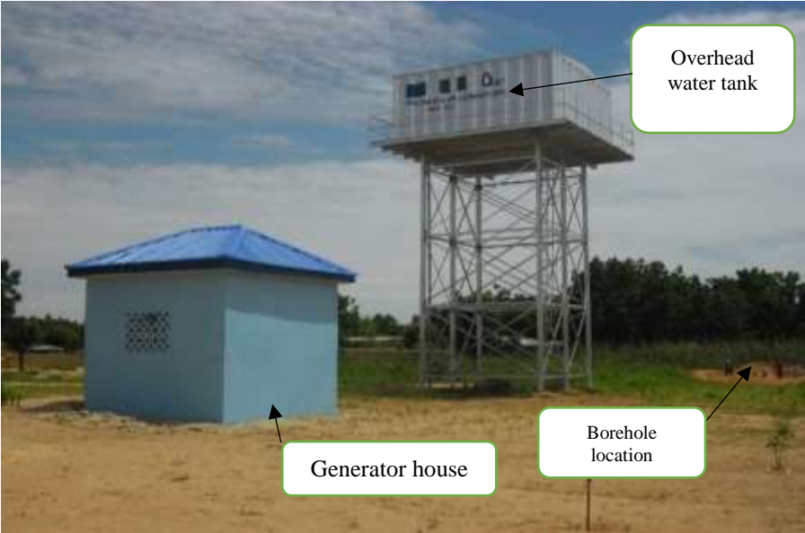
Figure 4.8: Small town water supply scheme
