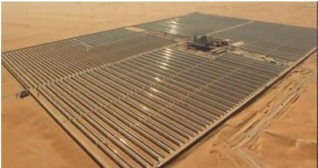
Figure 5-11 Shams1 Concentrated Solar Power Plant, Abu Dhabi (Source: Helioscsp Solar Thermal Energy News, 2014)
