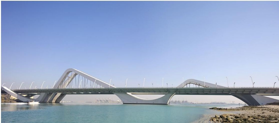
Figure 5-7 Sheikh Zayed Bridge, Abu Dhabi (Source: Hufton and Crow, 2014)
