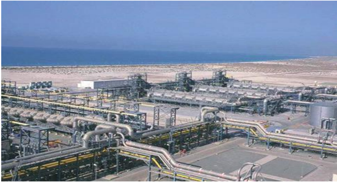
Figure 5-13 Al Taweelah B Desalination Plants, Abu Dhabi (Source: ACC, 2014)
