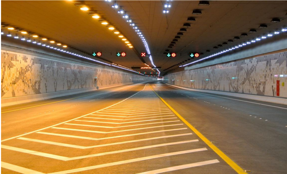
Figure 5-10 Sheikh Zayed Tunnel, Abu Dhabi (Source: SBD, 2014)
