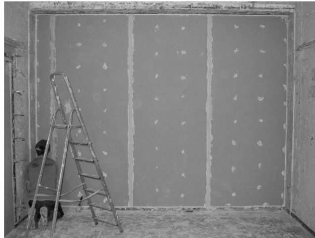
Figure 5. Mastic sealing on the metal-framed wall perimeter for the experimental test.
