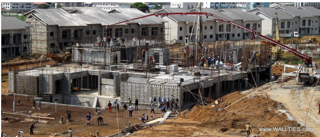
Figure 2.0: Typical Building Construction Project in Nigeria
