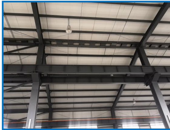
Fig. 1: Application of plate girders with stiffened webs in the laboratory of SWPU
