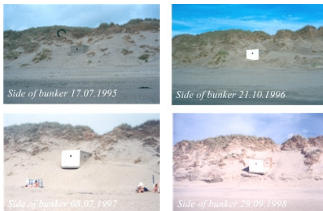
Fig. 3b. View from the south side of the bunker. Observe the exposure of the south-facing window and undercutting of the concrete platform
