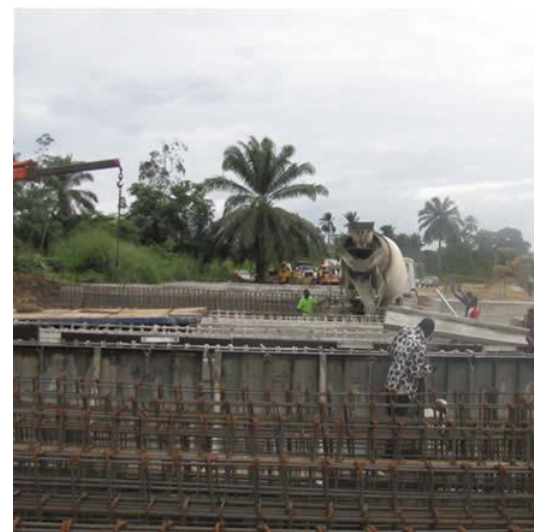
Figure 6.6 Construction of Bridge Piers
