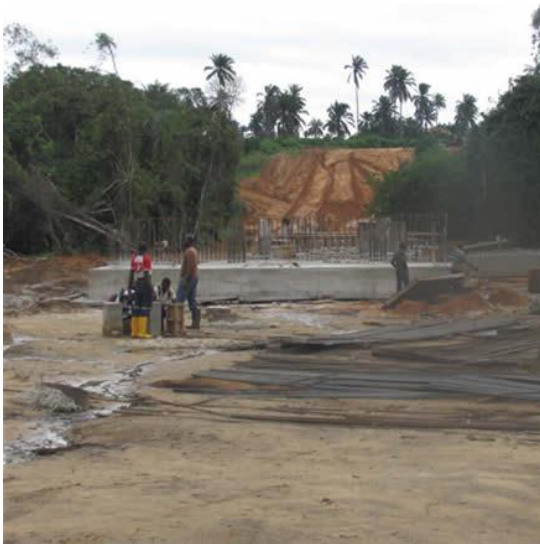
Figure 6.5 Construction of the bridge abutment
