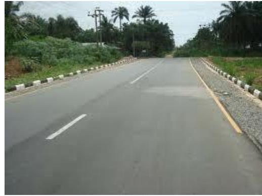
Figure 6.4 Finished road surface
