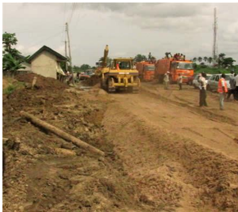
Figure 6.1 Clearing of the road
