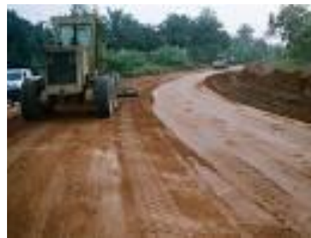
Figure 6.2 Grading of the road
