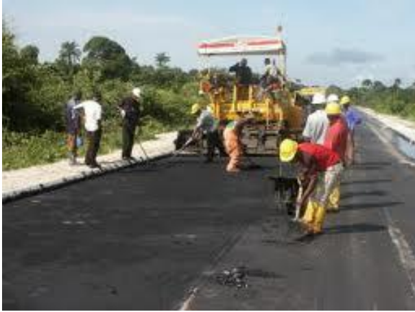
Figure 6.3 Asphalting of the road
