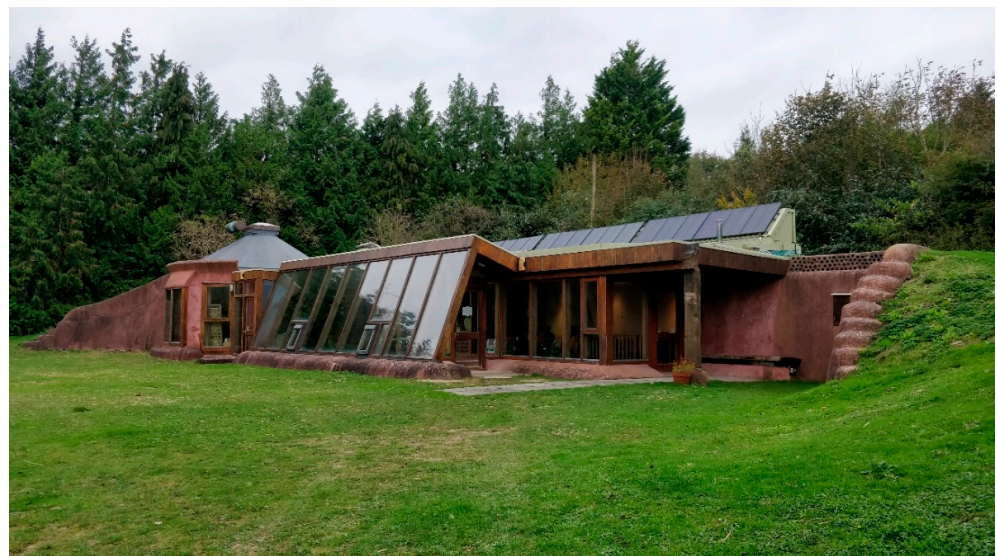
Figure 1. Photo of the Brighton Earthship (taken 03/11/2019) shows the south-facing glazing wall, angled for maximum solar gain, flanked by tire walls, and a roof that is topped with banks of photovoltaic solar panels.
